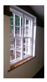
Made-to-Measure, White Powder-Coated aluminium frame Horizontal Sliding Secondary Glazing.
